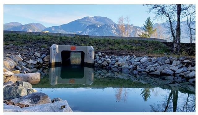
A box culvert installed in the dike to increase connectivity between the Squamish River and the estuary. (Credit: Edith Tobe)
